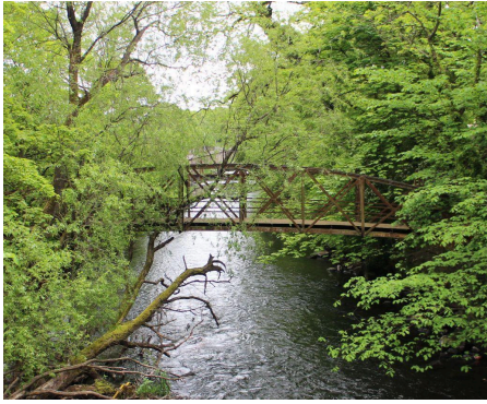
Kirkland Iron Bridge
